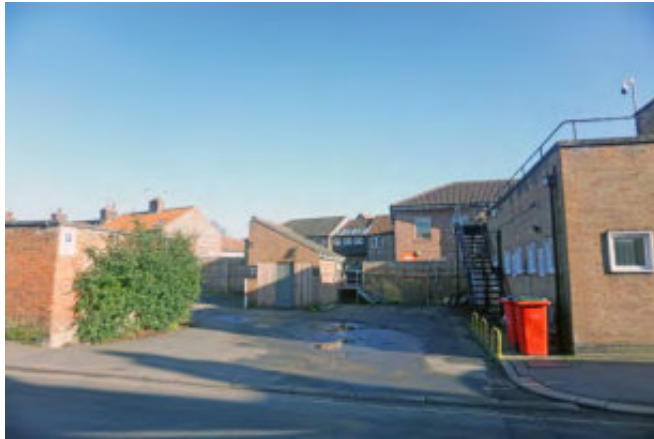
Poor quality service yard to the rear of Barclays
