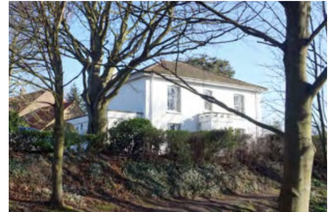
Early-twentieth century house adjacent to the Horn Pits proposed for inclusion within the Conservation Area boundary (area H on the plan)
