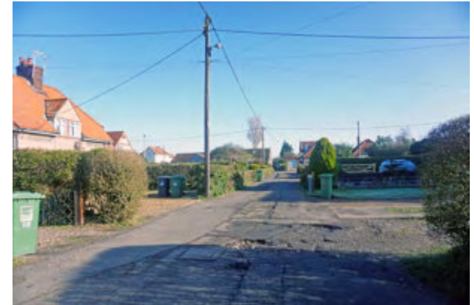
Poor surfacing of The Fairhaven
