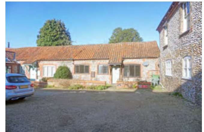
Converted outbuildings/stables off New Street
