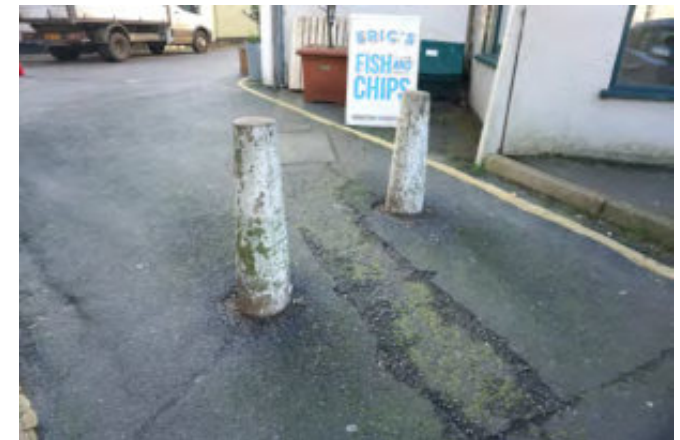
Unattractive concrete bollards on Fish Hill
