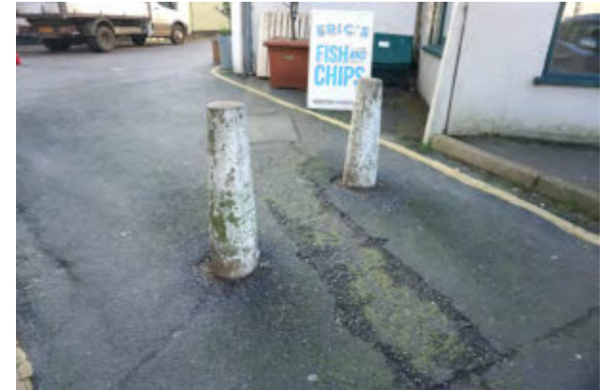
Unattractive concrete bollards with peeling paint
