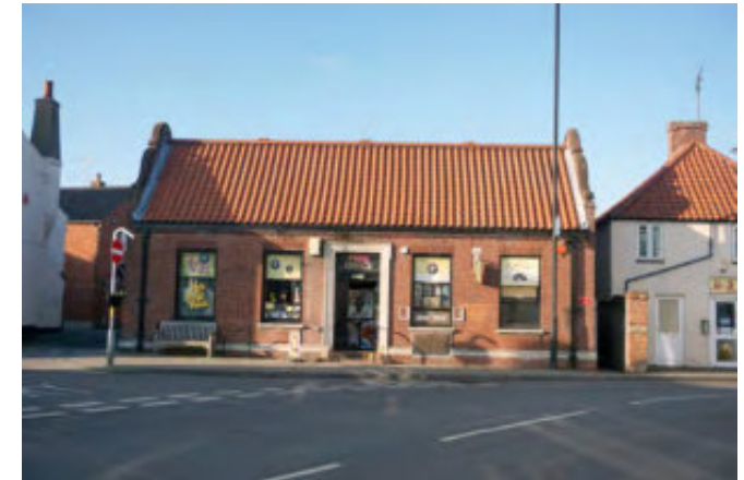
The former post office
