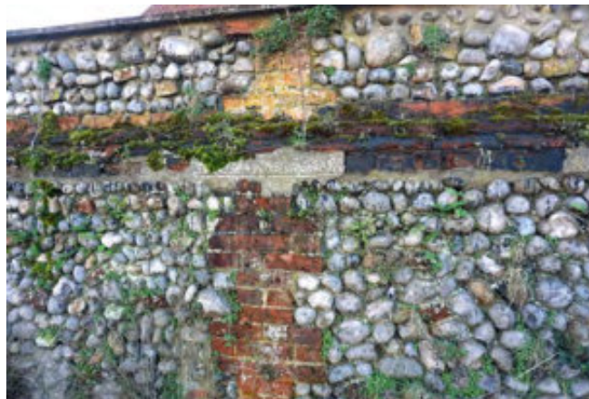
Wall with vegetation growth and patches of cement pointing, indicating damp and poor condition
