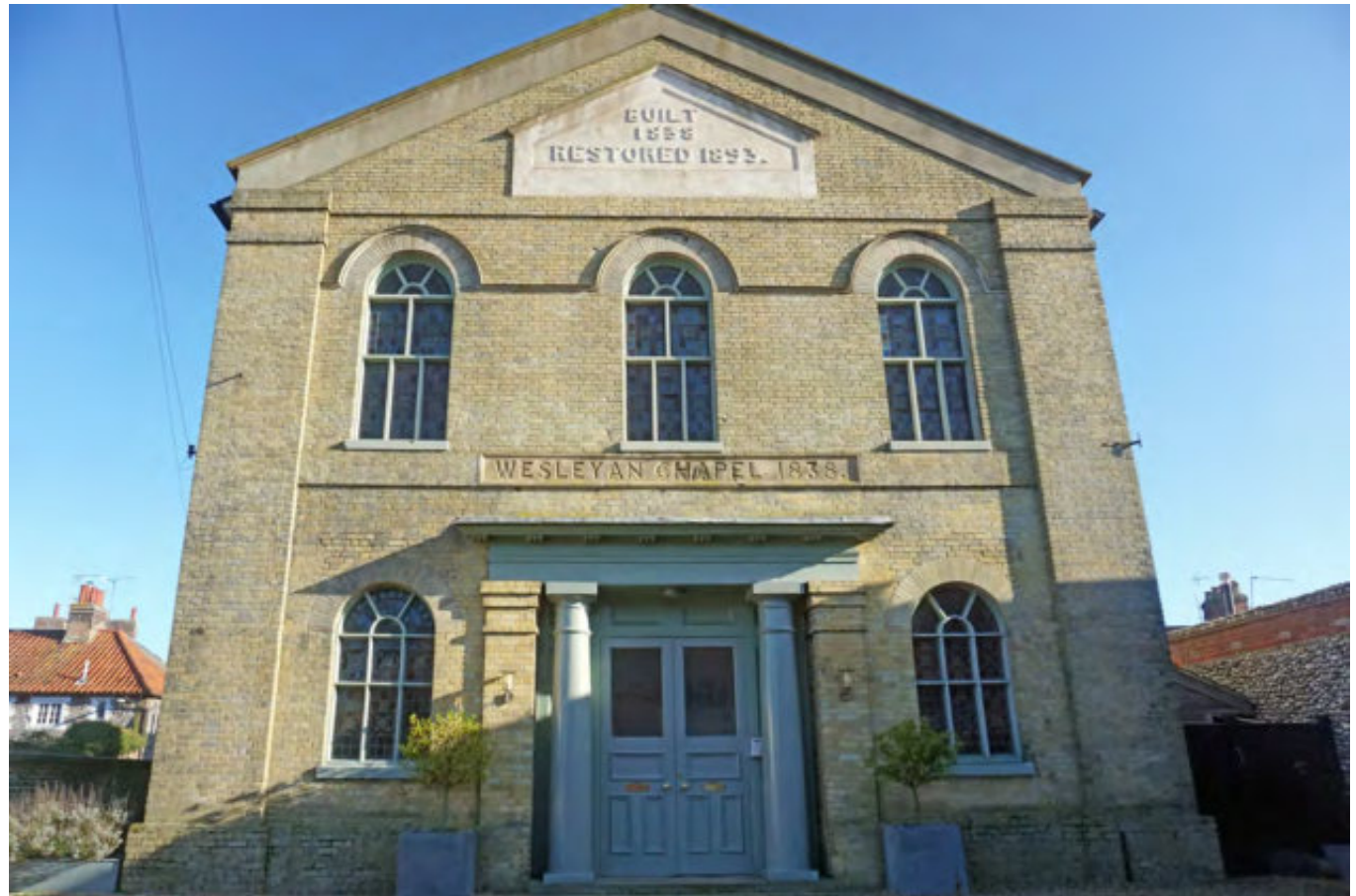
Wesleyan Chapel on New Street built 1838
