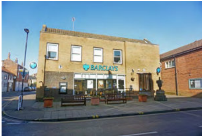
Barclays Bank, an unsympathetic building in the Conservation Area
