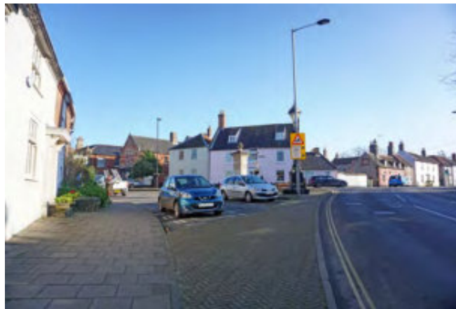
Parking and road signage at Obelisk Plain intrudes on the setting the historic obelisk and fountain/lamppost
