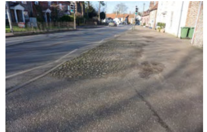
Cobbled areas to the pavements on Norwich Road
