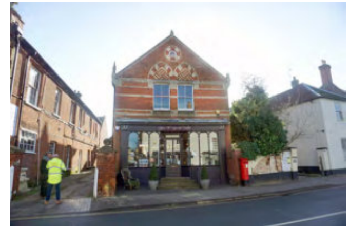
No. 33 High Street with unusual patterned brickwork
