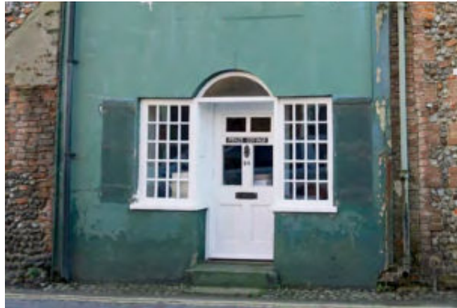
Poor condition of paintwork
