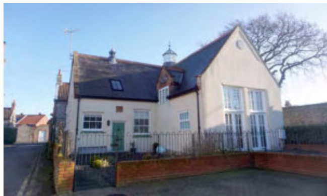
Former Country Primary School on New Road
