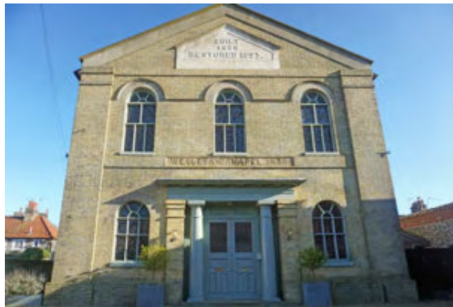
Converted Wesleyan Chapel on New Street
