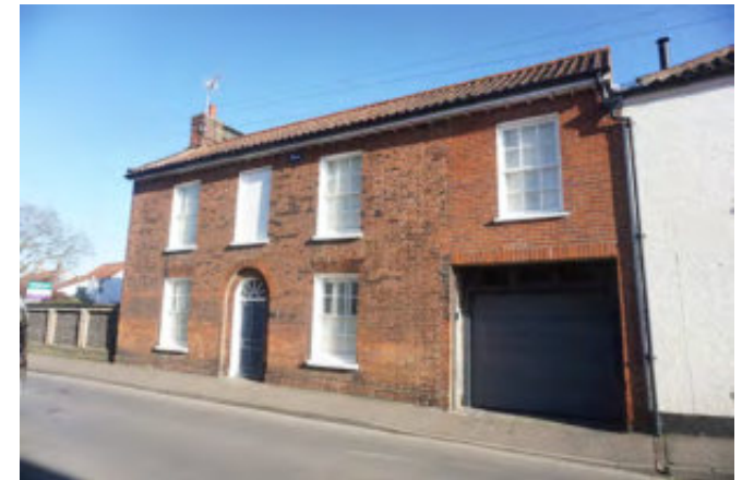
Unsympathetic garage attached to a listed building
